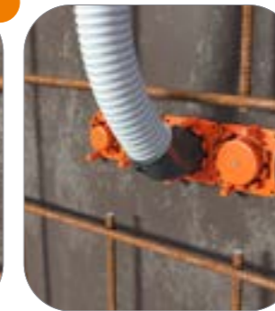
Nail the Front part to the formwork. The Front part can be firmly connected to other transitions and grommets thanks to the push-fit system. Push the transition onto the Front part. Ideal bending radius of 30°.
